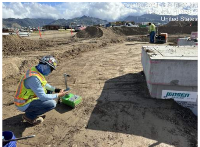
MPE performing compaction testing for the backfill around PB-9 on Pier 42
