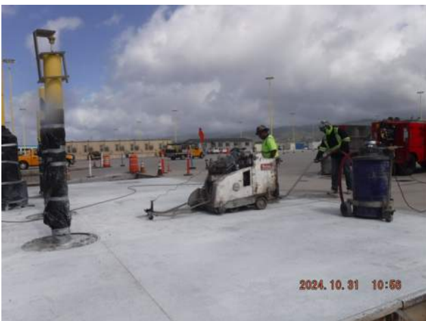
Pier 43: NCS crew on site to green saw cut the PCCP
