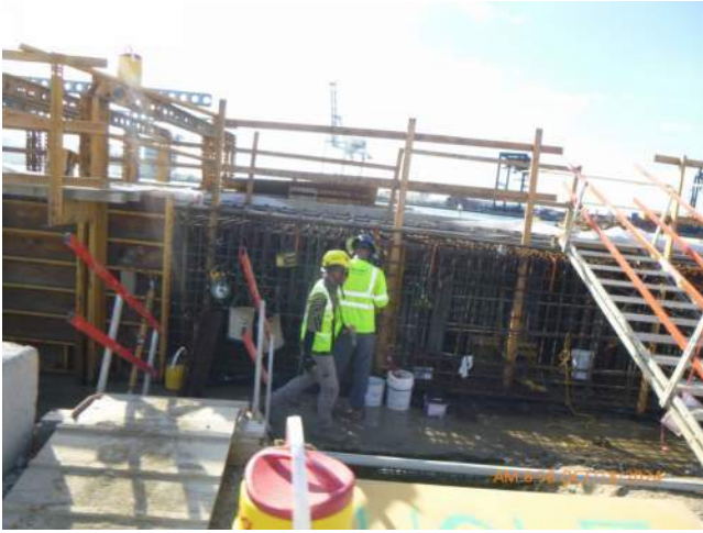
KIWC setting formwork for the WSCRb pour #A1 bulkhead.
