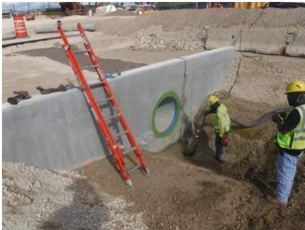
KIWC grinded and epoxied headwall penetration at P40F
