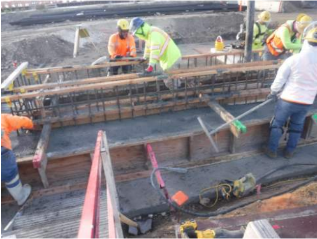
KIWC pouring concrete at TD2
