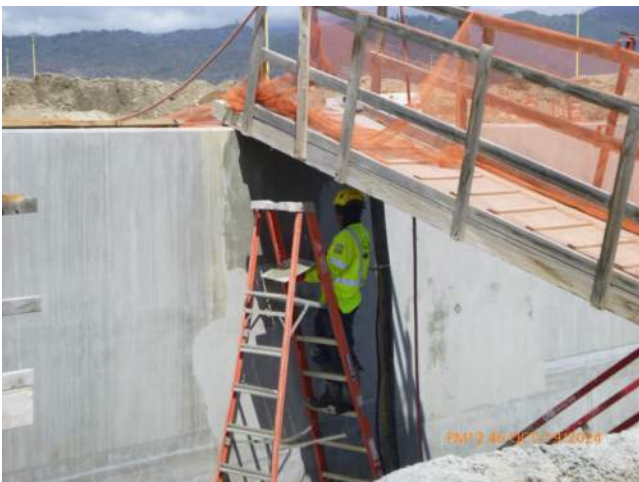
KIWC dry finishing the surface of the waterside of CWCB pour #23.
