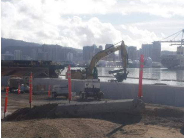
Excavator working at P43 Embankment
