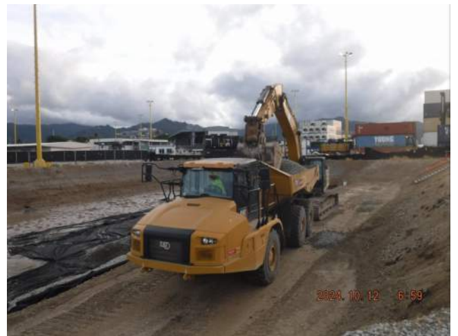
Pier 40F: Backfilled the dewatering pond
