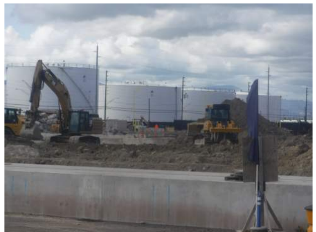
KIWC hauling and adjusting wet excavation material
