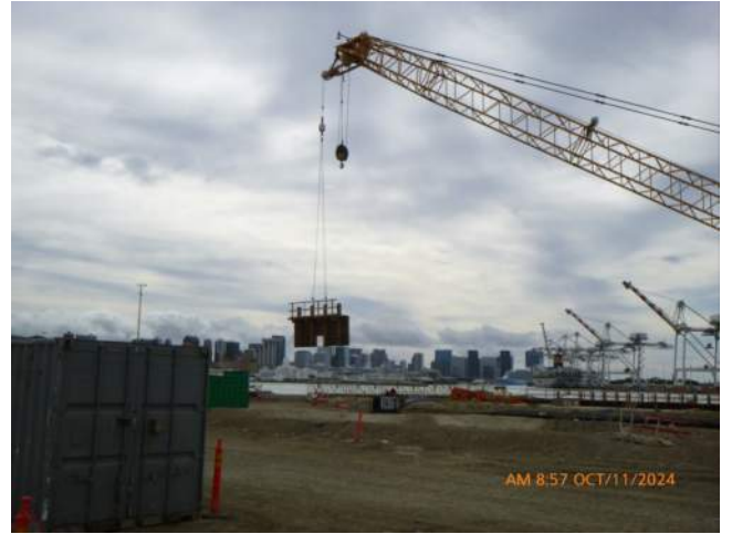
KIWC stripping formwork from around WSCRB pour #A1.
