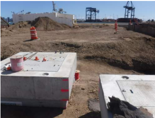
Pullbox #9 Trench Slope
