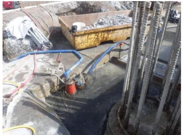
15-A4-36 and 16-A4-36 being chipped by KIWC
