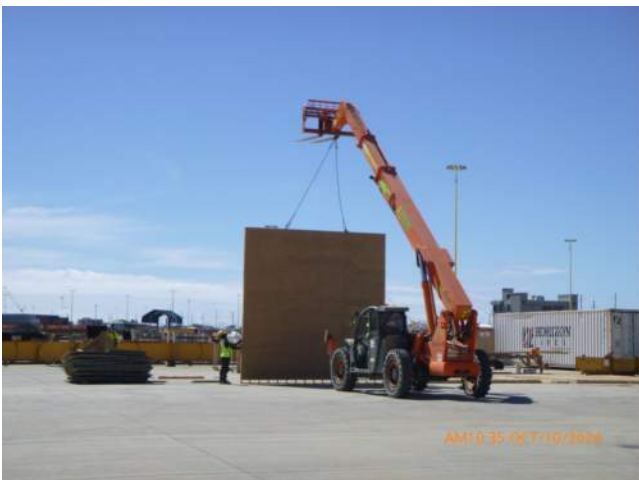
KIWC fabricating panels for dredging operation.
