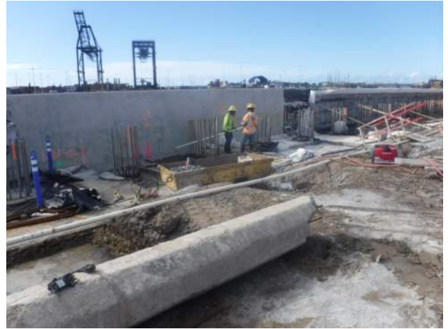
15-A4-36 and 16-A4-36 being chipped by KIWC
