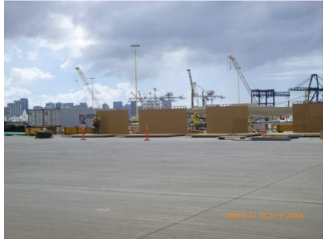
KIWC fabricating panels for dredging operation.
