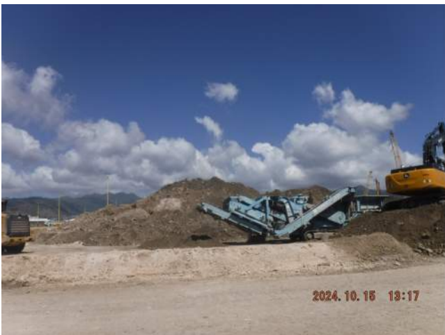
Pier 43: PFI resumed crushing the dredged material at the Pier 43 stockpile
