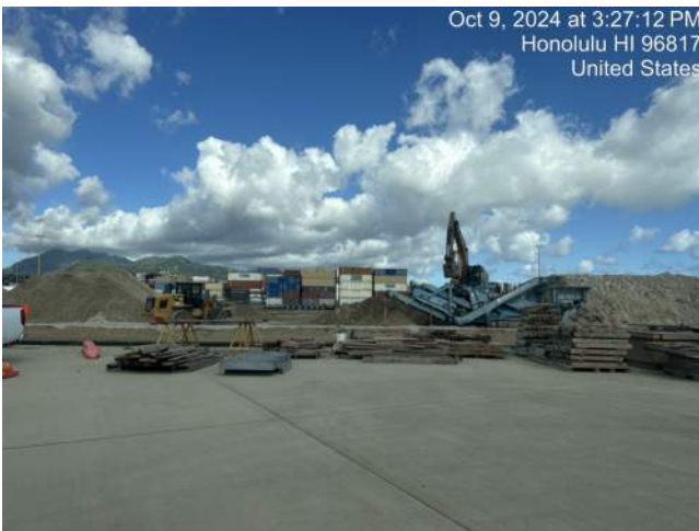
KIWC continued crushing dredge material with pineridge
