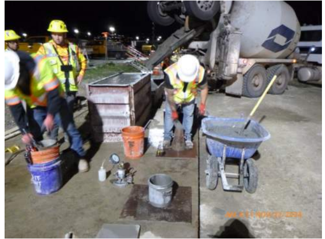
MPE testing delivered concrete for slump and air content.
