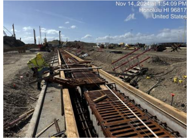
View of TD-2 installation progress on Pier 42
