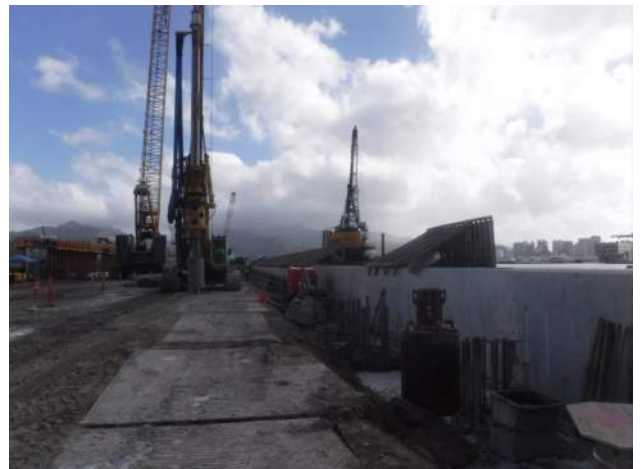
KIWC work at CIDH 6-A2-36
