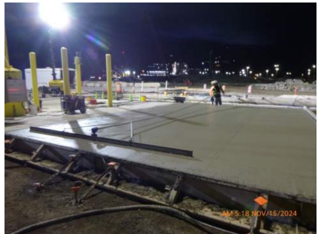
KIWC finishing the surface of the paving pour.
