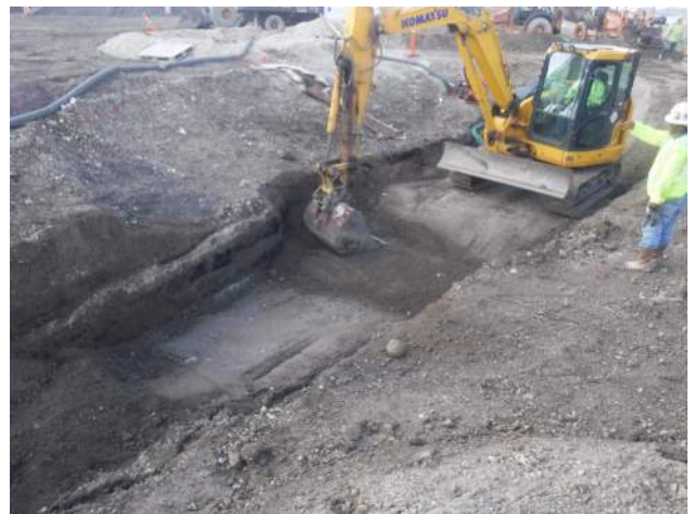
PE backfilling and compacting PB9/LSCRB Connection
