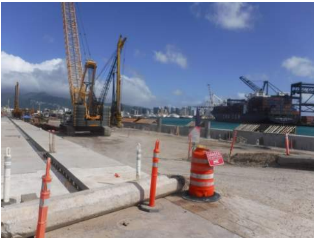
KIWC work at P43 preparing to drill and pour CIDH
