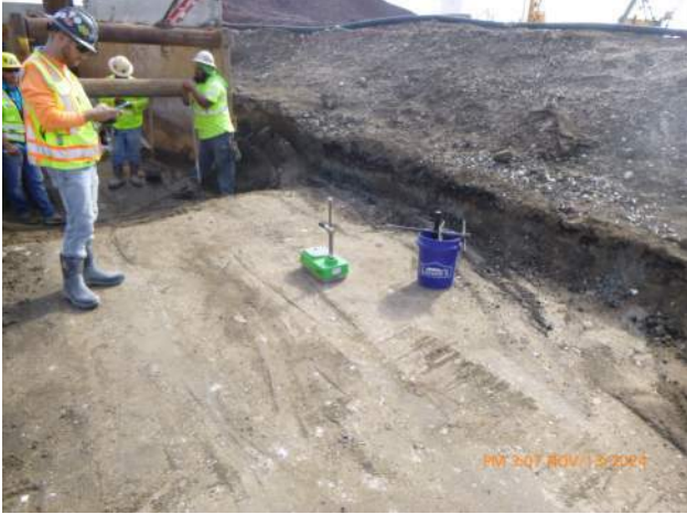
MPE testing compacted backfill over ductbank on pier 42.
