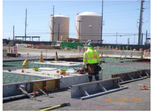
KIWC setting formwork around the WL 12 manhole blockouts.
