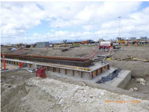
HRSPI set rebar for the TD-2 rebar cage.
