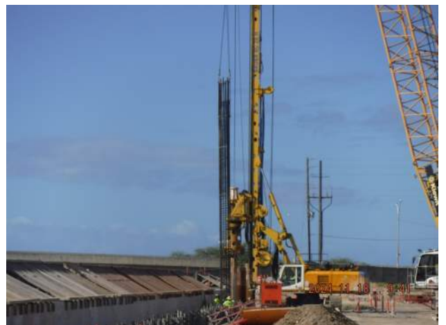
Pier 43: KIWC Foundation installing the rebar cage in CIDH 6-A2-36
