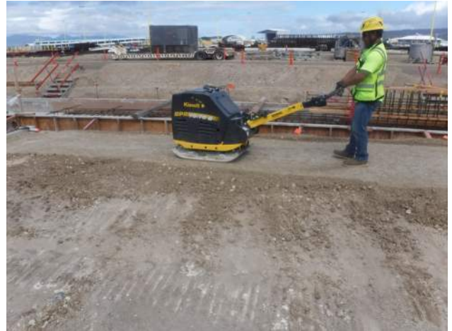
KIWC compacting backfill at SD-4
