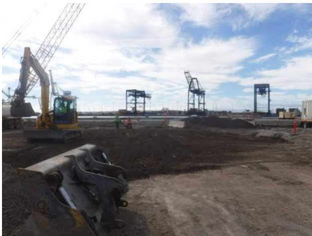
PE backfilling and compacting at LSCRB Connection
