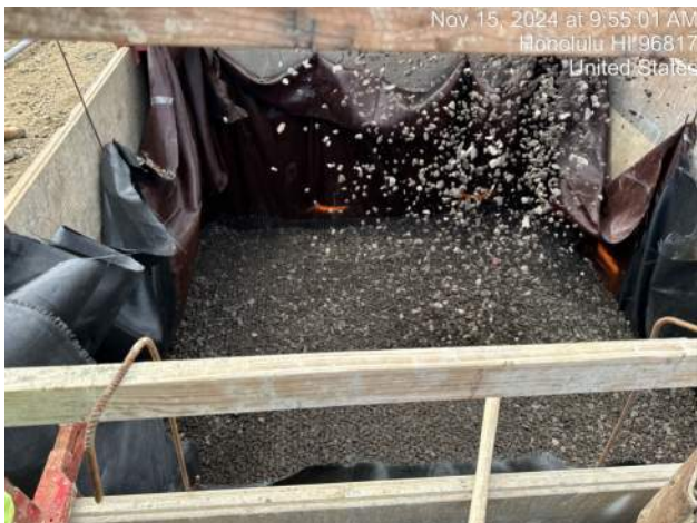
PECL progress installing the stabilized layer for PB-15 on Pier 41
