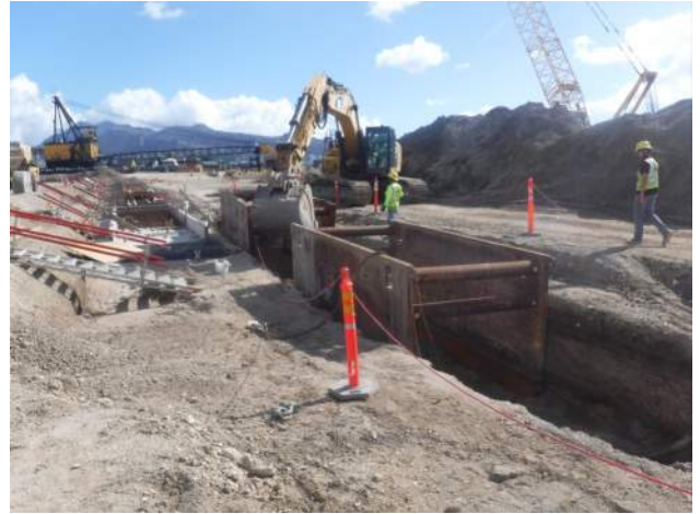
KIWC preparing to pull out shoring from SD-4.
