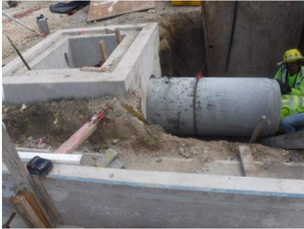
KIWC installing 24" RCP at SD-4.
