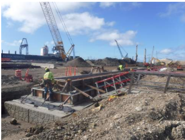
KIWC securing outer wall forms at TD2
