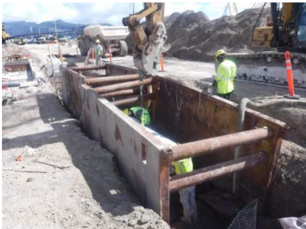
KIWC installing 24" RCP into SD-4.
