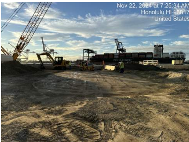
PECL compacting lift 14 of the PB-9 to LSCRB area on Pier 42
