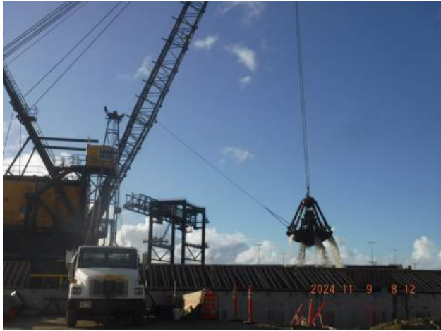
Pier 43: KIWC DB Seattle continued in water dredging from STA 7+00 to STA 6+00
