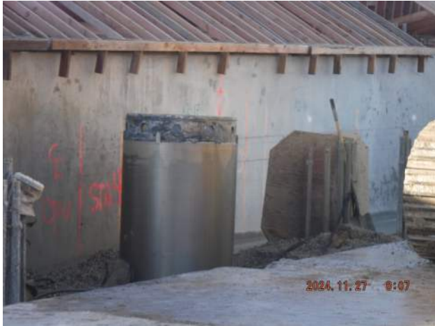
Pier 43: KIWC foundation crew pulled out the casings from CIDH 18-A2-36
