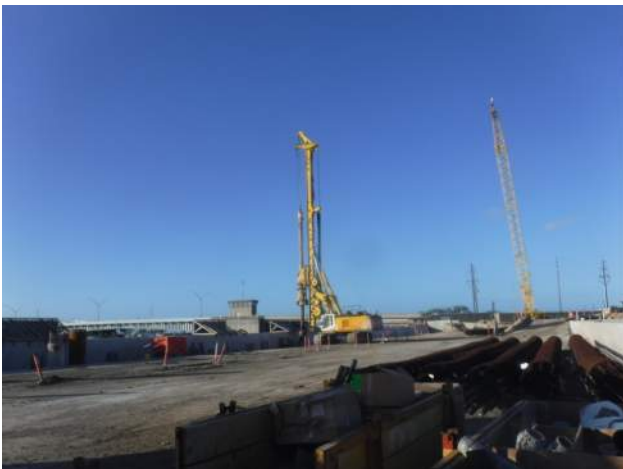
KIWC work at P43 drilling CIDH
