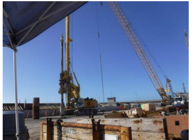
KIWC work at P43 removing shaft casings.
