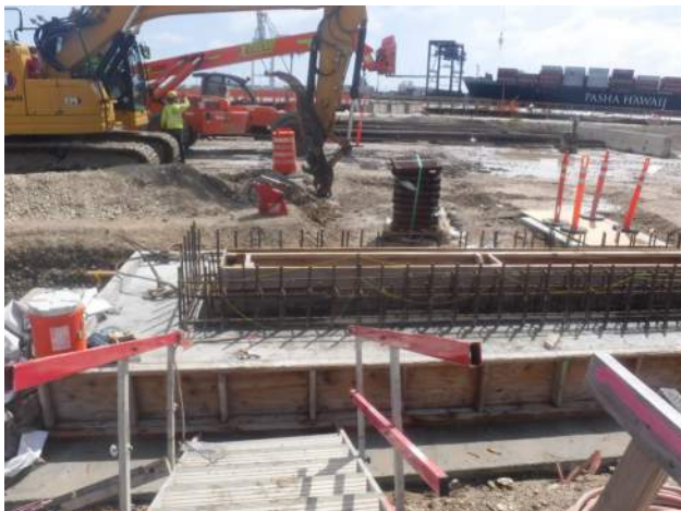
KIWC preparing to install Trench Grate and Frames
