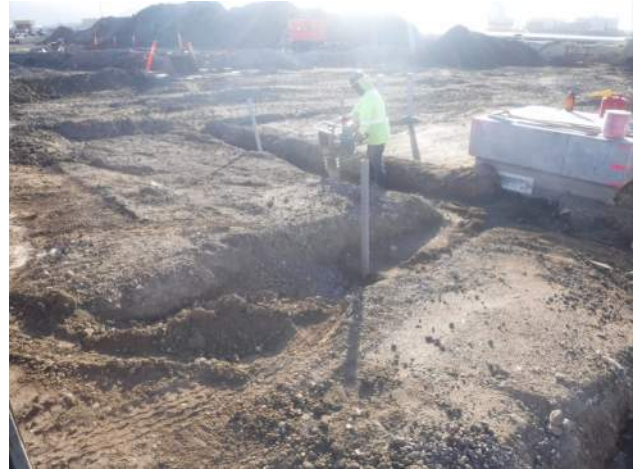
PE compaction and backfill at PB9
