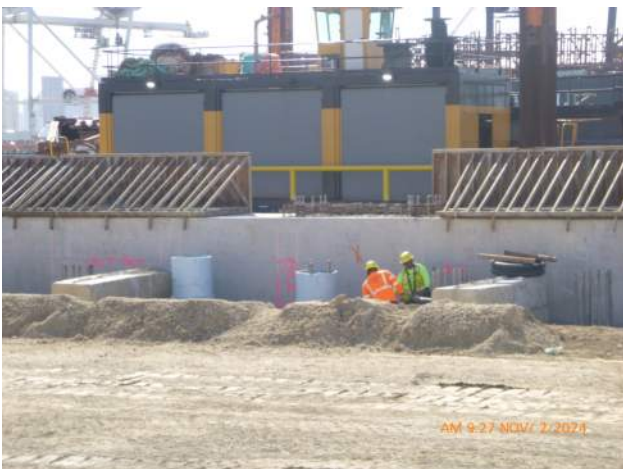
KIWC constructing an equipment pad around CIDH shaft 15-A2S-36.
