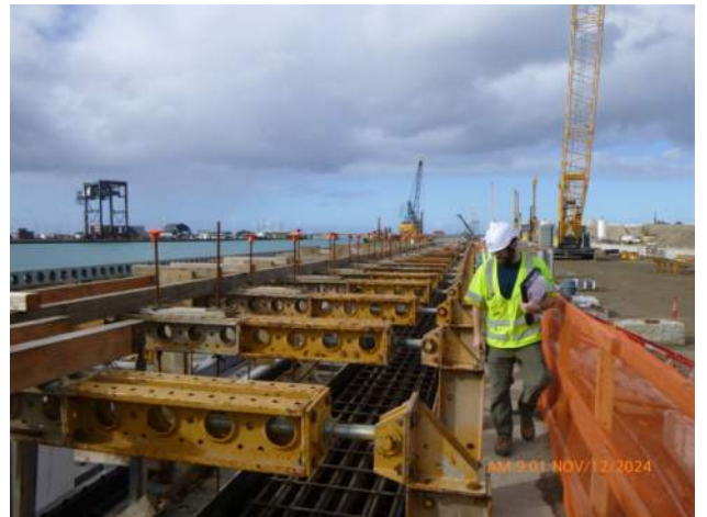
MN performing a structural observation for WSCRB pour #A1.
