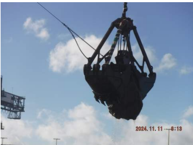
Pier 43: KIWC DB Seattle continued in water dredging from STA 7+00 to 6+00
