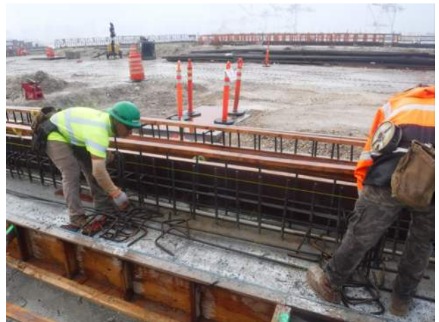
HRSPI installing horizontal rebar reinforcements and U-bars.
