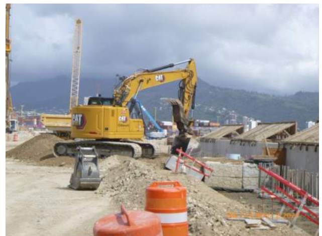
KIWC moving 36" CIDH cages to the staging area on pier 43.
