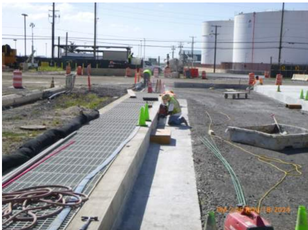
KIWC grinding off the existing waterproofing from TD-3.
