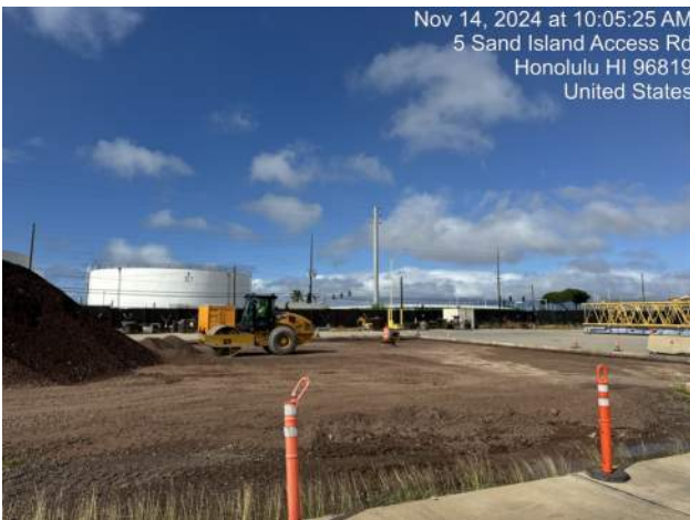
KIWC continued method compaction for the KIWC maintenance area
