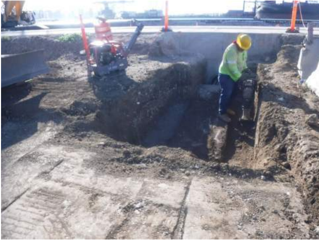
PE compacting and backfilling at Ductbank @ LSCRB
