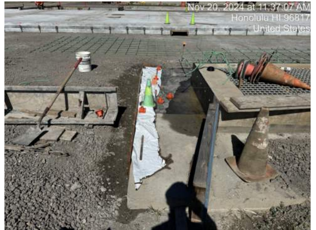
KIWC performed spall repair for the west end of TD-3
