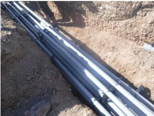
Pier 41: PE laying conduit pipes at PBC/PBE-15.
