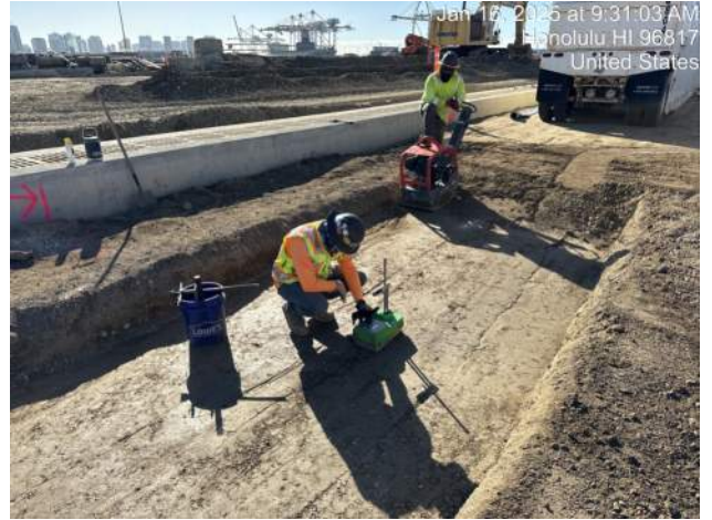
MPE performing compaction testing for PE backfill on Pier 41
