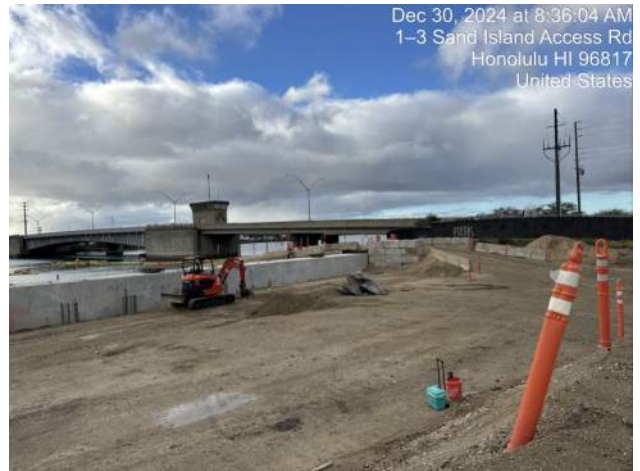
KIWC performing prep for the WSCRb mud mat on Pier 43
