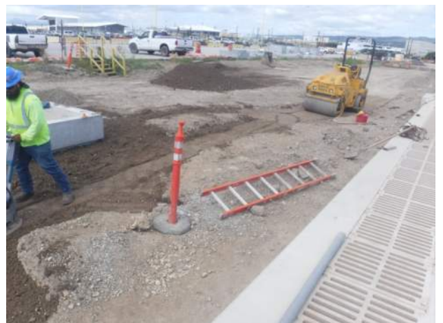
PE compacting at PBC-15.
