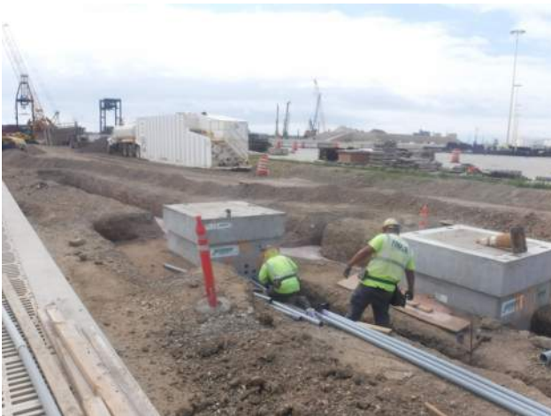
PE installed conduit pipes north of PBC-15
