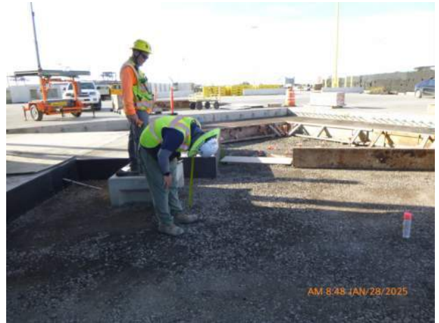
KIWC performing grade check on the MT-9 paving breakout.
