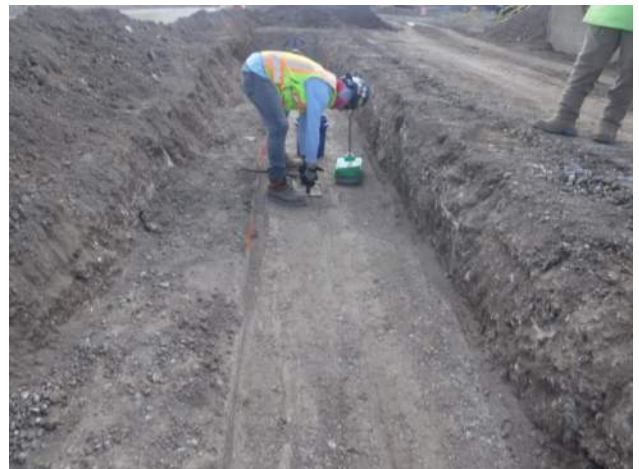
MPE testing backfill compaction test at TD-1
