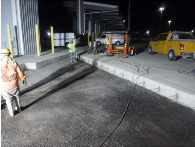
KIWC epoxying and doweling at Pasha Maintenance Blockout
