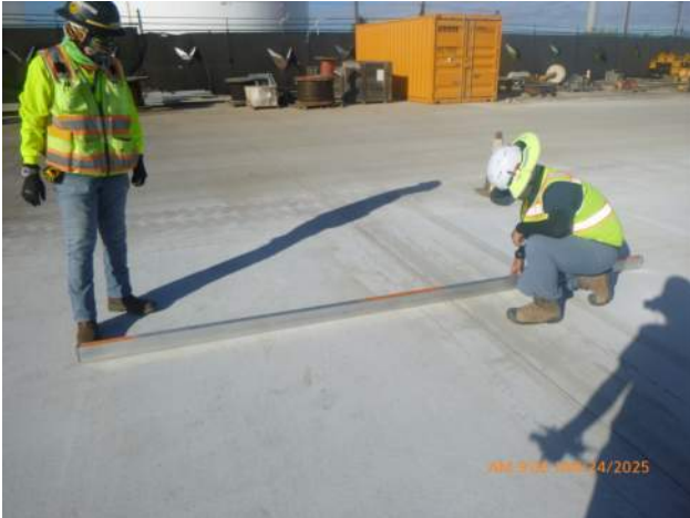
YKE straightedge testing the MT-3 PCCP paving blockout.
