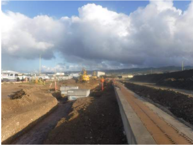
PE conducting backfill and compaction at PBC-15 north.
