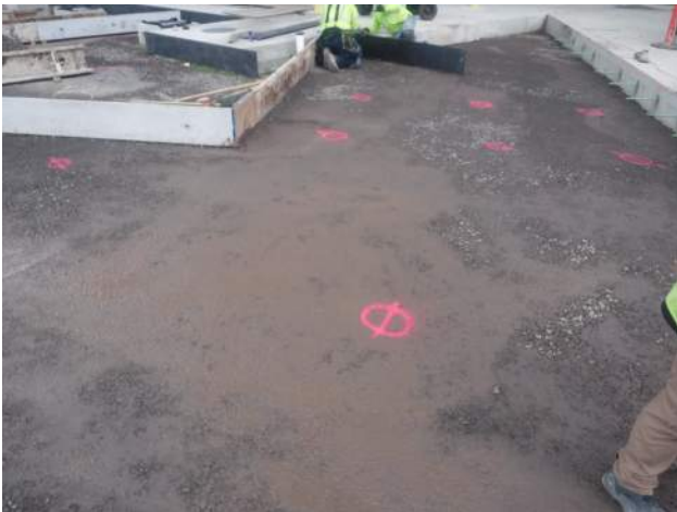
KIWC performing grade check at MT-9.
