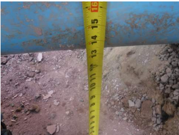
PE chipping off concrete jacket to get clearance between waterline
