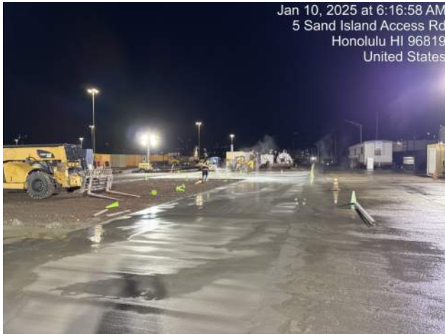
KIWC spraying curing compound over MT-3
