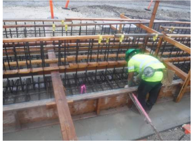
HRSPI fixing splice issue at TD-2 P5.
