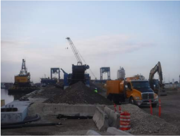
KIWC crushing dredging spoils at P41.
