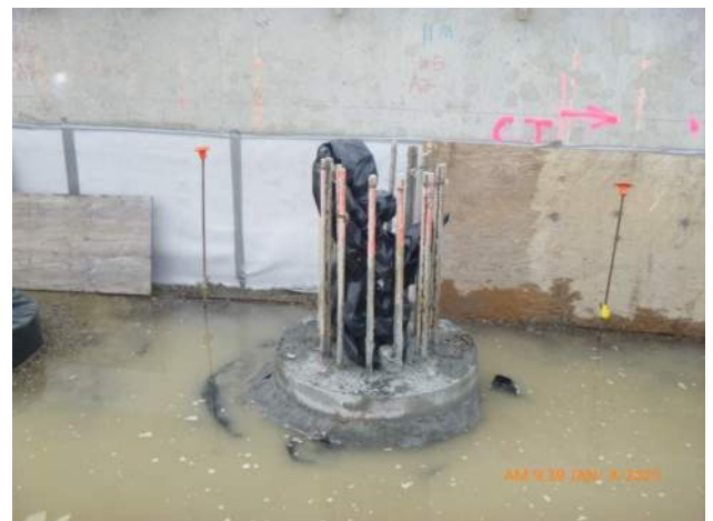
View of CIDH shaft with excess concrete removed.
