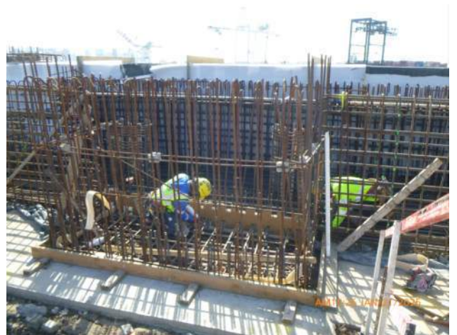
KIWC installing formwork around the CPV in WSCRB pour #A5.
