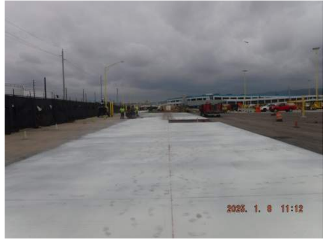
PCCP: MT 5 was sprayed with J9 concrete curing compound
