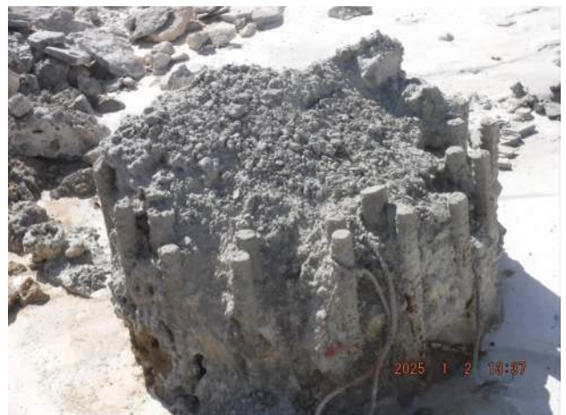
Pier 42: Existing condition of the CIDH piers in the junction structure
