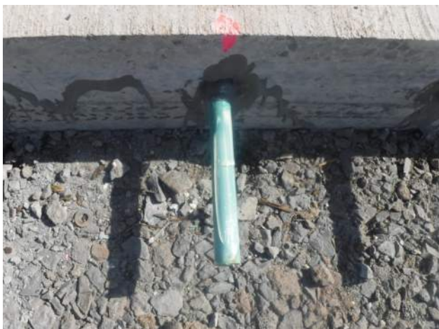
PCCP: Paving crew applied grease of the dowels
