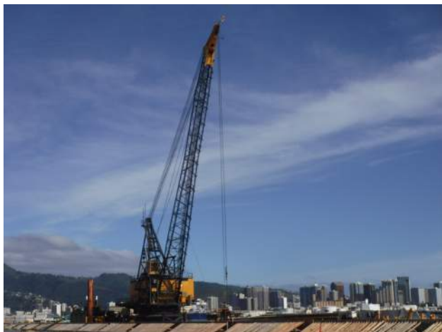
Pier 43: KIWC DB Seattle continued water dredging between STA 5+00 and STA 7+00
