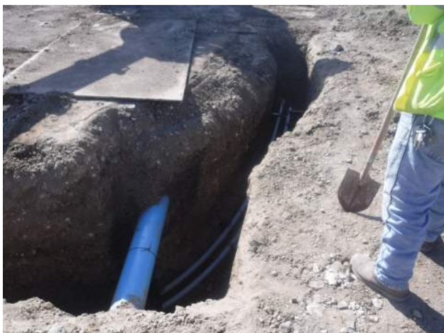
PE installing conduits west of PBC-15.
