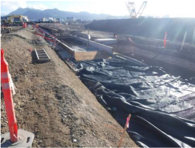
KIWC preparing to install mud mat forms at TD-2.
