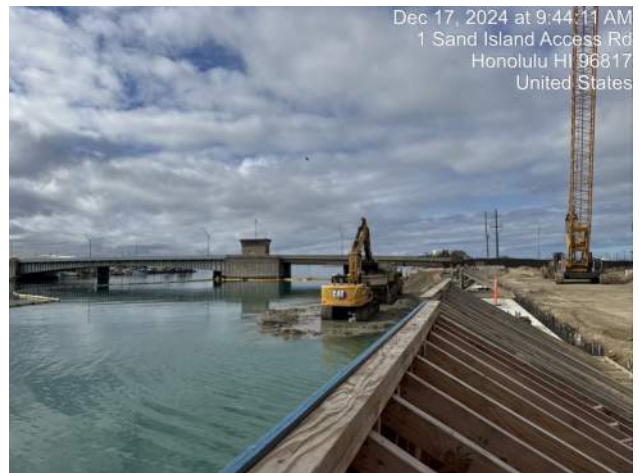
KIWC performing landside dredging on Pier 43
