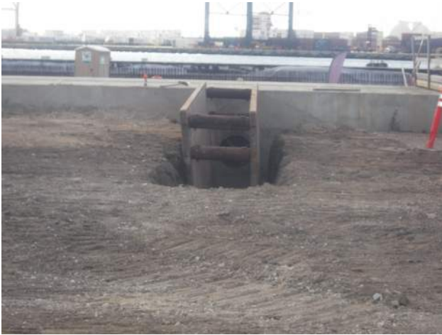
KIWC installed shoring at SD-5A.
