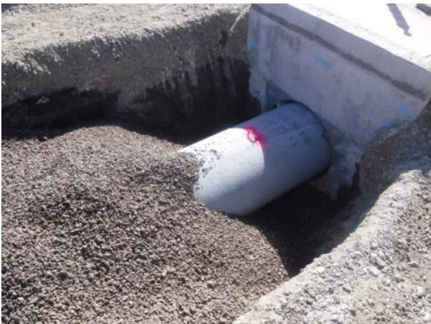
KIWC cut and covering at SD-4
