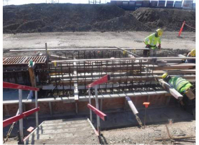
KIWC installed templates and waterstops at TD-2 P5
