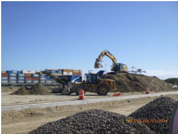
KIWC crushing dredged spoils on pier 41.
