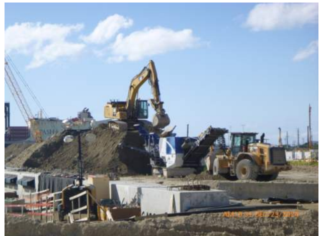
KIWC crushing dredged spoils on pier 41.
