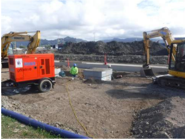
PE backfilling and compacting at PB-15
