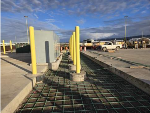
HECO Block out: HRSPI crew installed rebar mat
