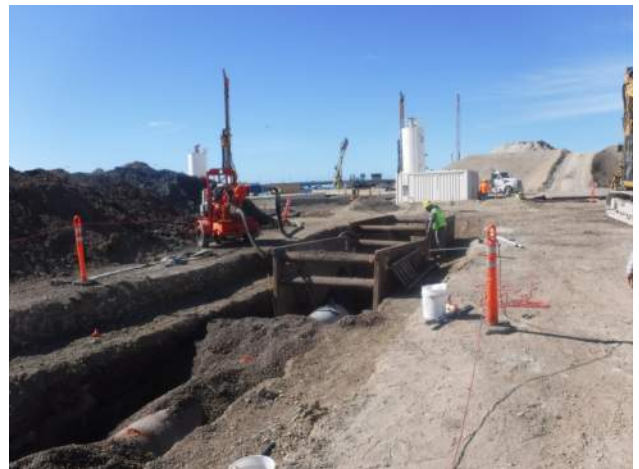
KIWC cut and covering at SD-4
