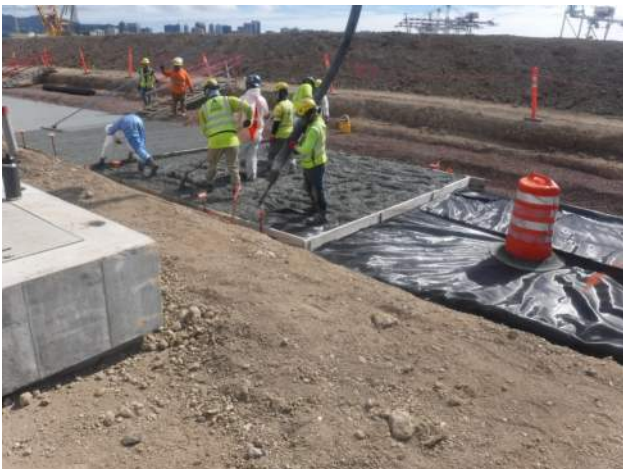
KIWC placing mud mat at TD-2 P5/P4.
