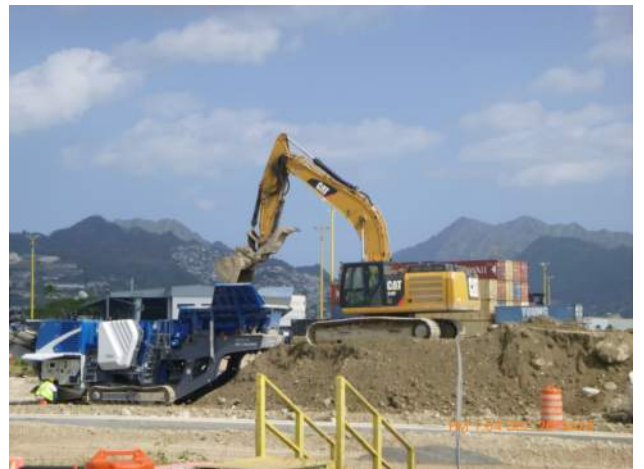
KIWC crushing dredge spoils on pier 41.
