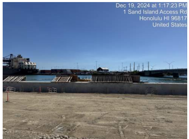
KIWC continued landside dredging at approximate Sta. 1+50 to 1+00
