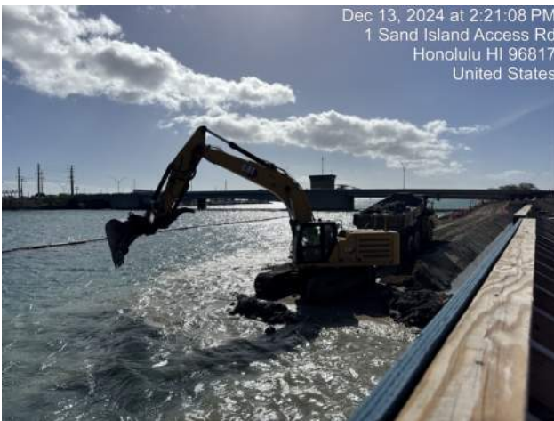
View of landside dredging on Pier 43
