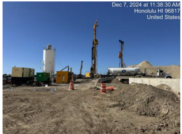
View of PF continuing soil mixing at the junction structure area
