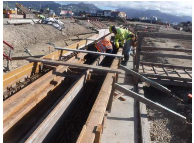
KIWC measuring levels and elevation at TD-2.
