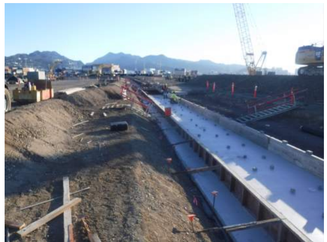
KIWC installing dobies and chamfers at TD-2.
