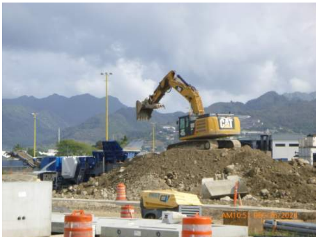
KIWC crushing dredge spoils on pier 41.
