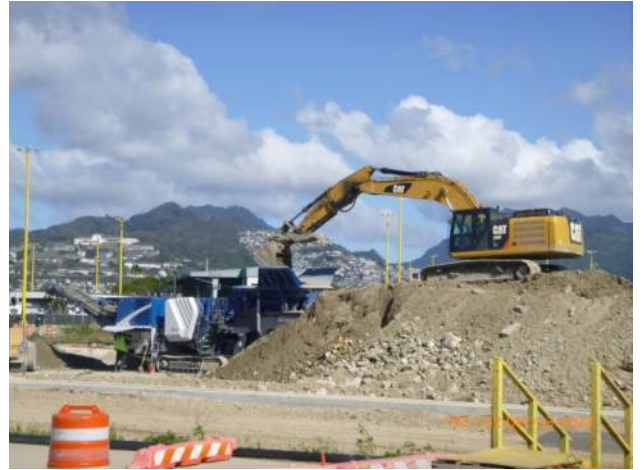
KIWC crushing dredged spoils on pier 41.
