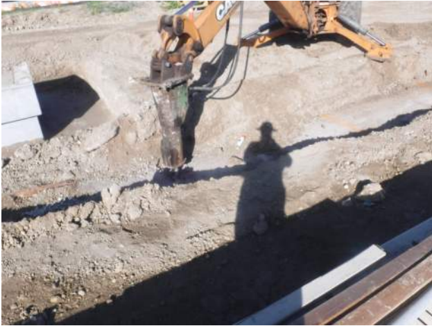
PE demolishes ductbank east of PBE/PBC-15.
