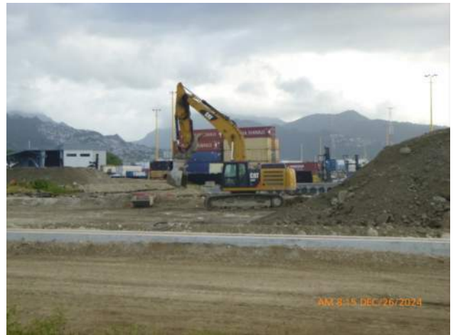
KIWC crushing dredge spoils on pier 41.
