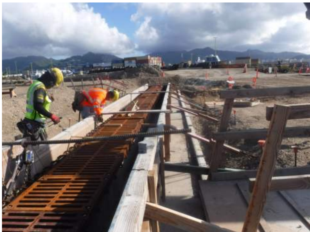
KIWC adjusted and lifted rebar at TD-2.
