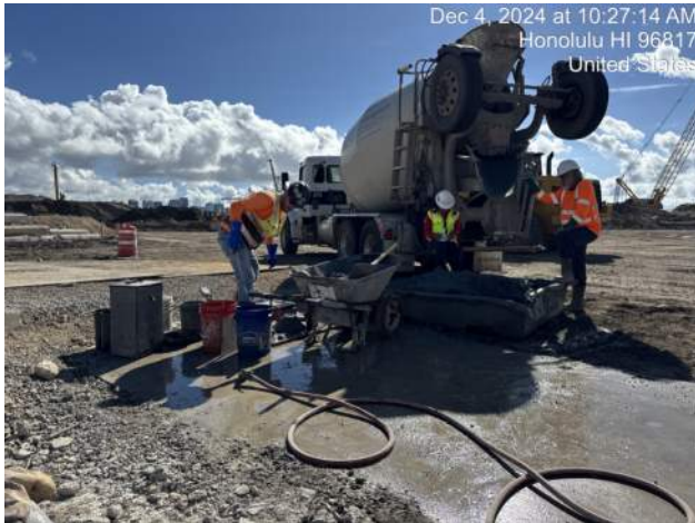
MPE performing concrete testing for truck 2 of the CIDH pour
