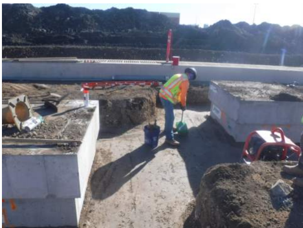
MPE testing backfill and compaction at PB-15.
