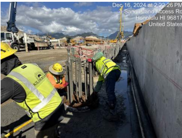
KIWC finished pouring shaft 21-A1-36
