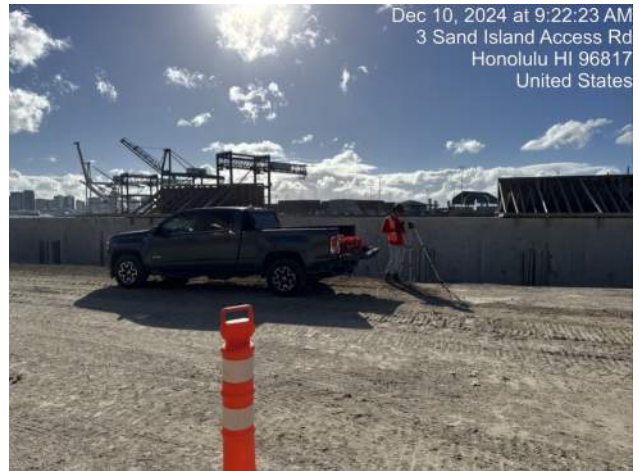
AFT performing CSL testing for shaft 30-A1-36
