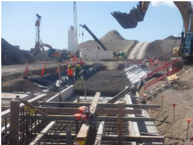
KIWC installing stabilization layer at TD-2.
