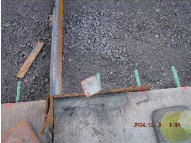
PCCP: KIWC mason crew continued spall repair of the PCCP
