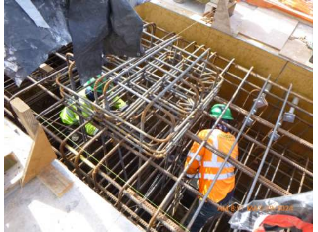
HRSPI setting rebar for the marine bollards in capping beam pour #20.
