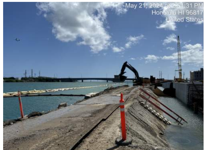
KIWC continued waterside dredging at Snug Harbor
