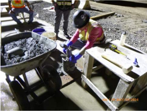
MPE testing delivered concrete for air content.
