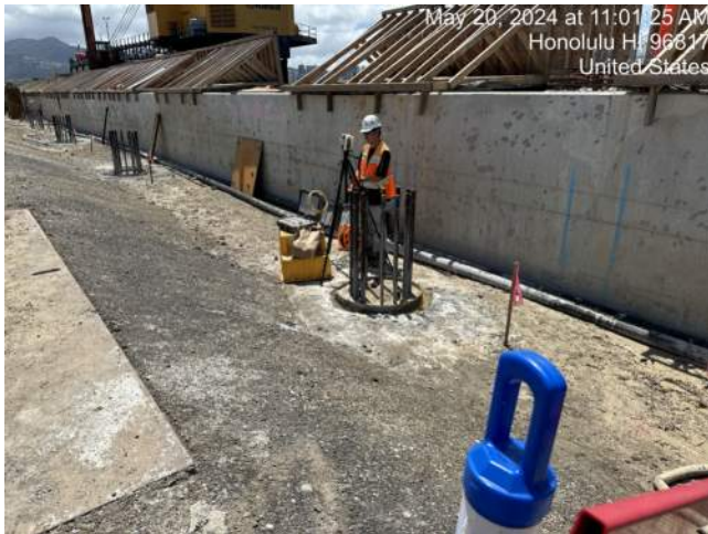
AFT performing CSL testing for 5 CIDH shafts this shift
