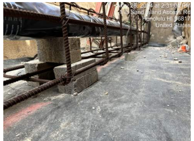
View of the poly wrap and bottom cover of the DIP for the W-2 siphon
