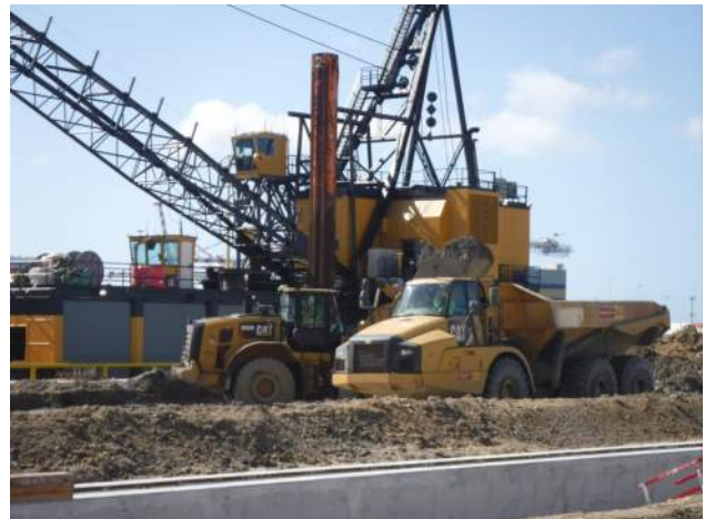
Pier 41: The dredged material is hauled out to Pier 43 stock pile
