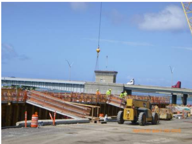
KIWC installing formwork for capping beam pour #20.
