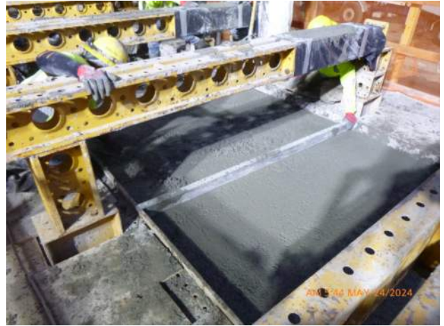
KIWC finishing the surface of capping beam pour #19.
