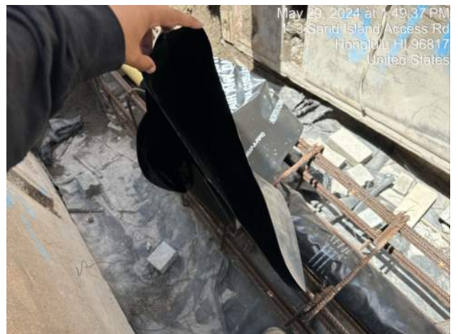
View of the polywrap for the DIP installation for W-2
