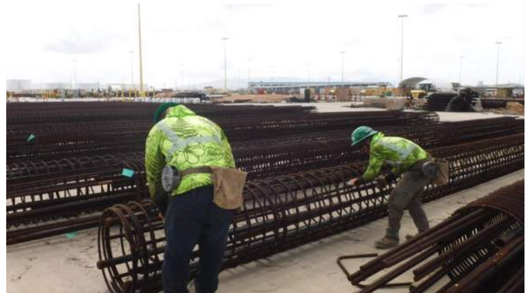
PCCP: HRSPI correcting the rebar laps for the 36-inch rebar cages
