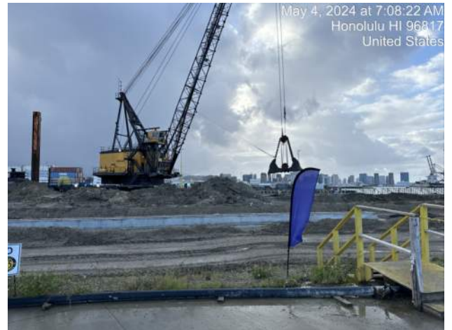
KIWC continued in-water dredging on Pier 41
