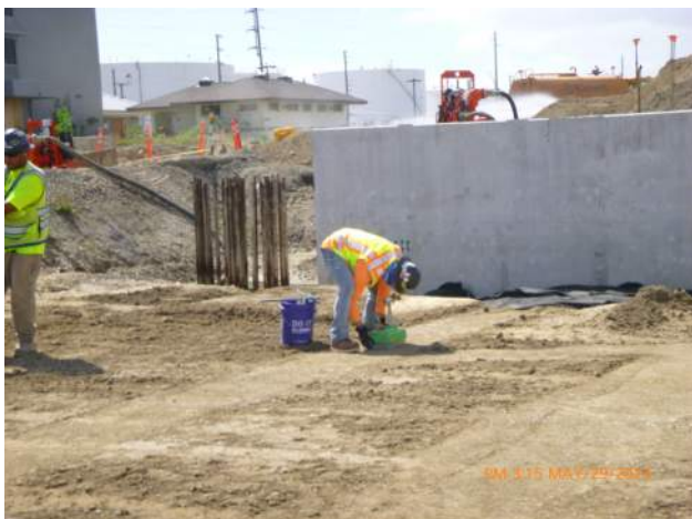
MPE performing compaction testing for tie rod backfill.
