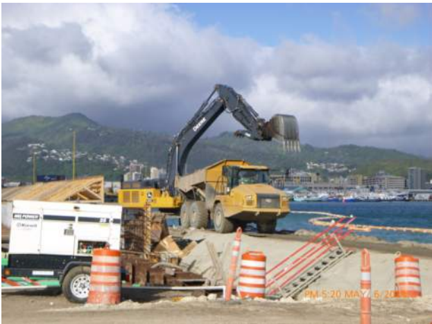
KIWC performing on-land dredging along pier 42.
