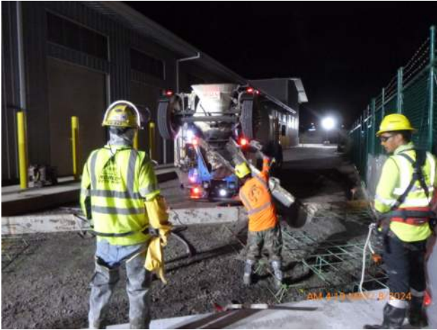
KIWC pouring the PCCP blockout near the maintenance building.
