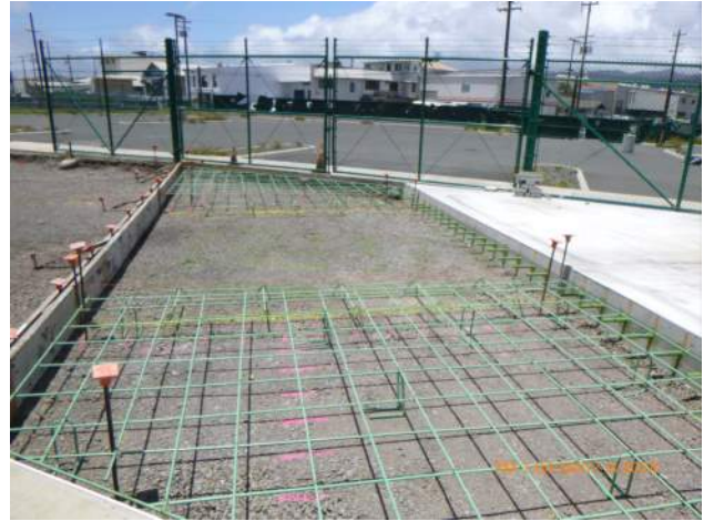
View of PCCP blockout near the maintenance building.
