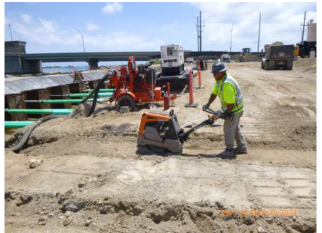
KIWC backfilling and compacting over tie rods on pier 43.
