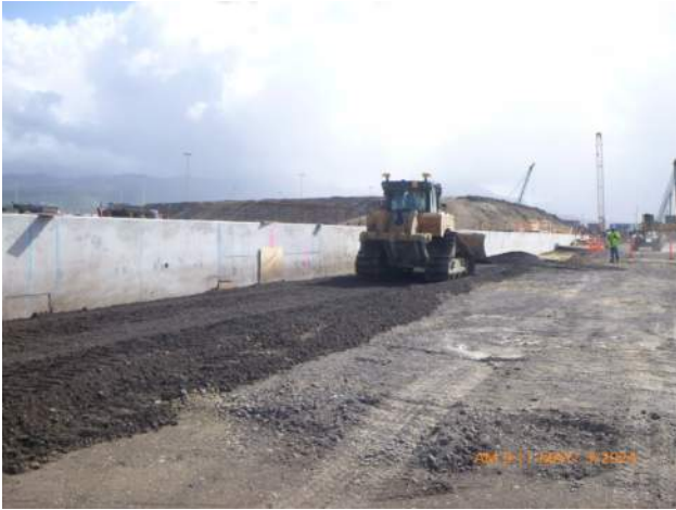
KIWC backfilling on the waterside of the LSCRB on pier 43.
