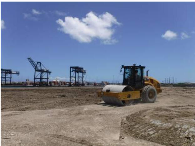
Snug Harbor: The CAT CS 56 vibratory roller was used to compact the dredged material over the surcharge (18th fill)
