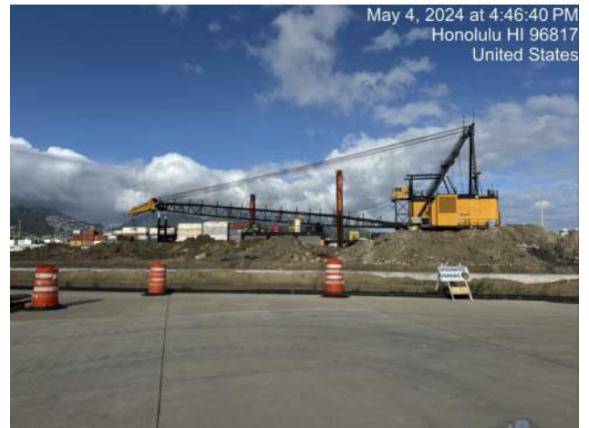
KIWC finished dredging for the shift
