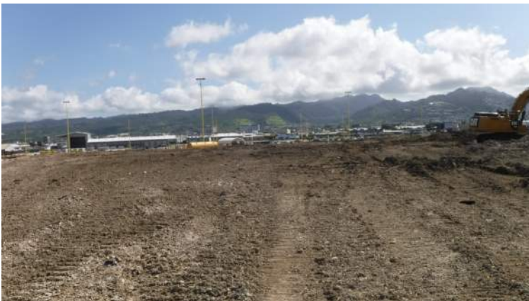
Snug Harbor: KIWC civil crew continued to use the CAT 336 excavator to spread the dredged material over the surcharge
