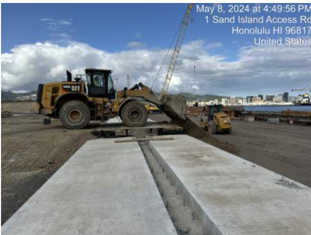
KIWC constructing the vehicle ramp over the LSCRB on Pier 43
