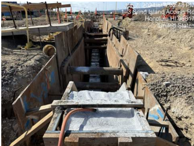
KIWC finished pouring the W-2 RCJ and setup the curing system
