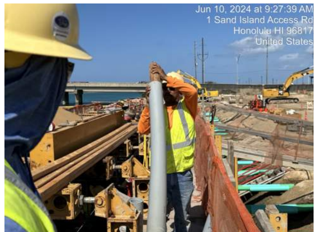
PE using the 3.5" diameter mandrel to test the 4" conduit
