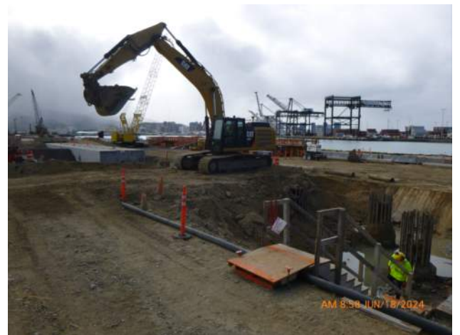
KIWC excavating around CIDH shafts for the pier 43 LSCRB on pier 43.
