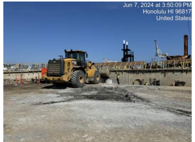
KIWC placing 3B fine material into the hole after KIWC reached the lap splice section of the remaining shaft 58-A4-36
