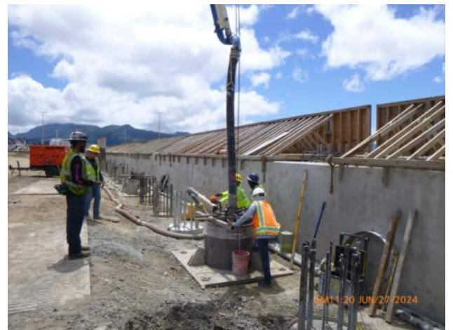
KIWC pouring concrete into CIDH shaft 37-A4-36.
