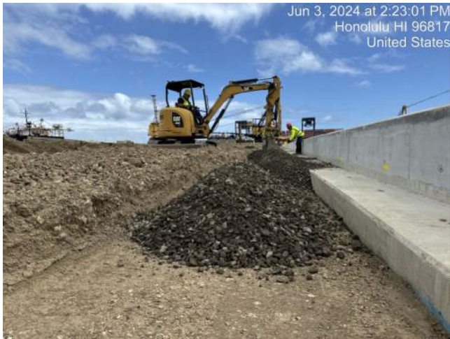
KIWC backfilling the waterside of trench drain 3 on Pier 41
