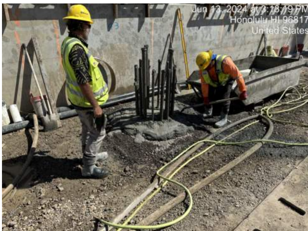
View of shaft 43-A4-36 after pulling the casing
