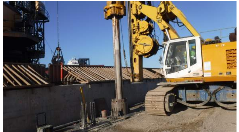
Pier 42: KIWC Foundation crew resumed drilling CIDH #31-A4-36
