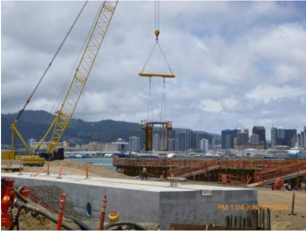
KIWC stripping formwork from capping beam pour #19.
