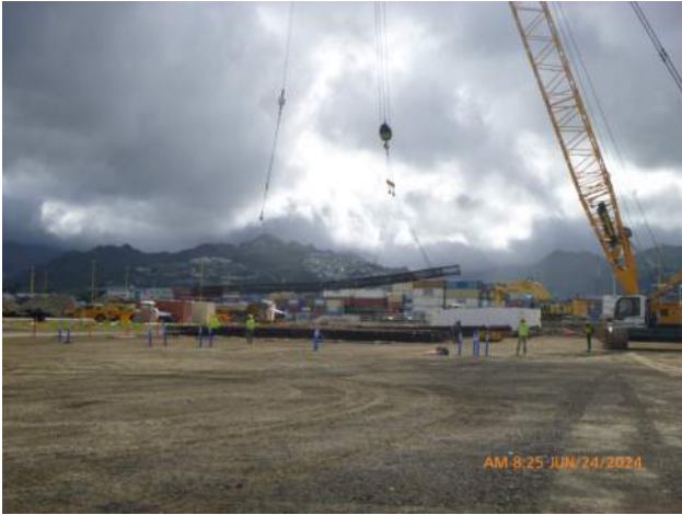
KIWC setting 36" CIDH rebar cages using the Liebherr crane.
