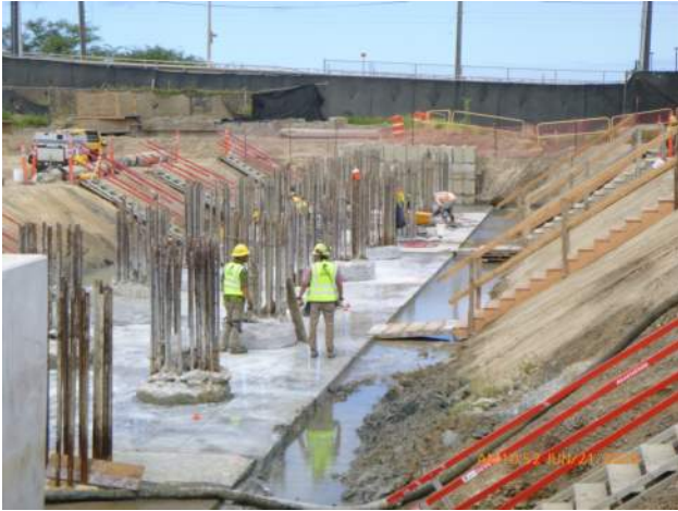
KIWC chipping down CIDH shafts to top elevation on pier 43.
