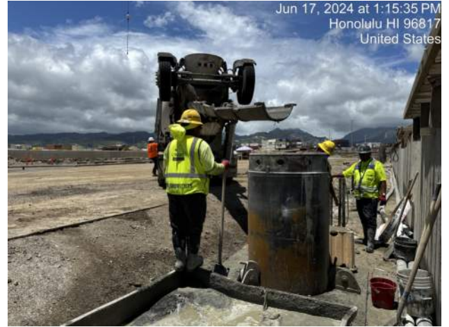
KIWC topping off location 31-A4-36 on Pier 42
