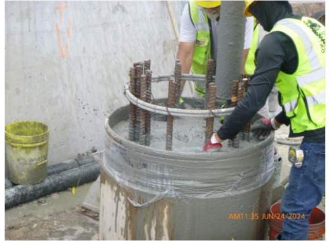
KIWC pouring concrete into CIDH shaft 27-A4-36.
