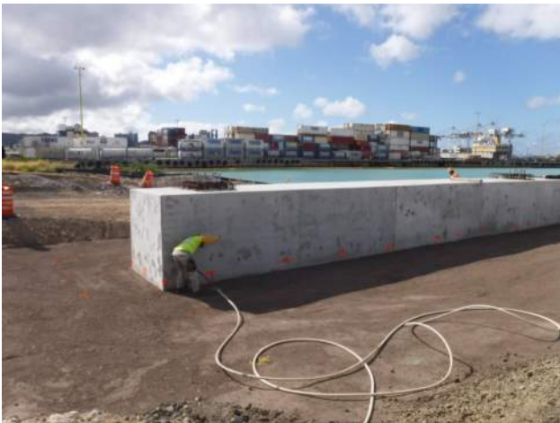
Pier 41: KIWC mason crew grouted the form tie holes of P1 of the CWCB
