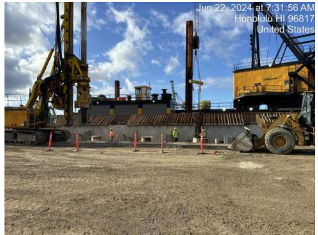
KIWC placing a rebar cage into location 23-A4-36 on Pier 42
