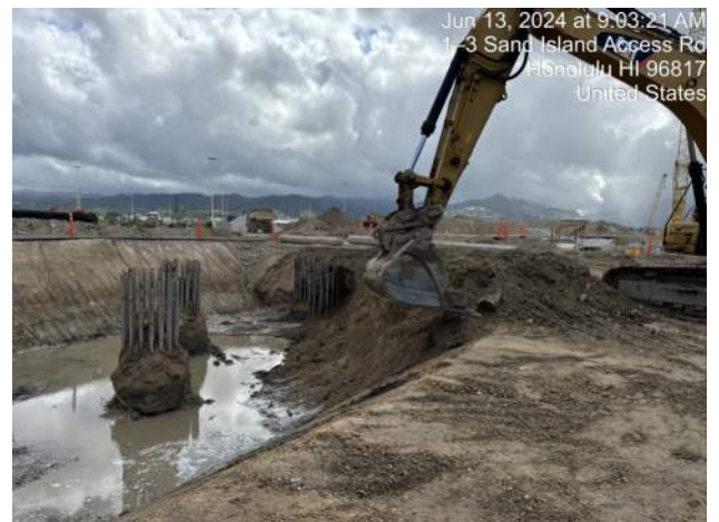
KIWC continued excavating for P8 of the LSCR on Pier 43
