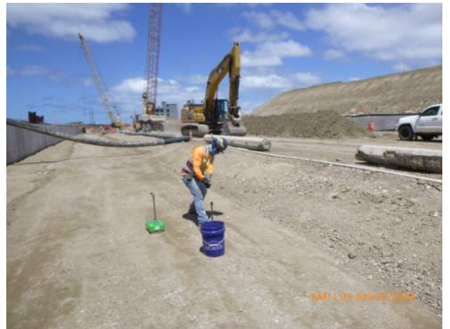
MPE performing compaction tests on the CWCB backfill.
