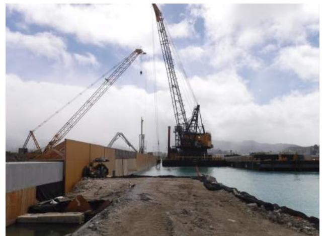
Pier 42: KIWC DB Seattle continued in water dredging
