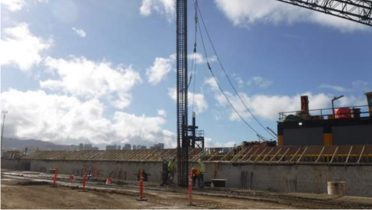
Pier 42: KIWC foundation crew installing the rebar cage for CIDH # 46-A4-36
