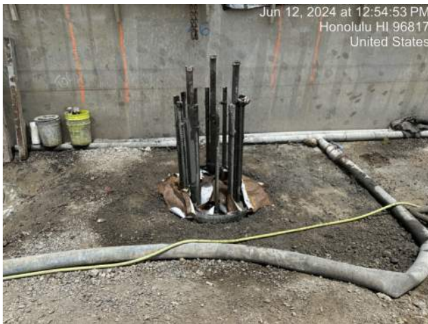
KIWC curing shaft location 46-A4-36
