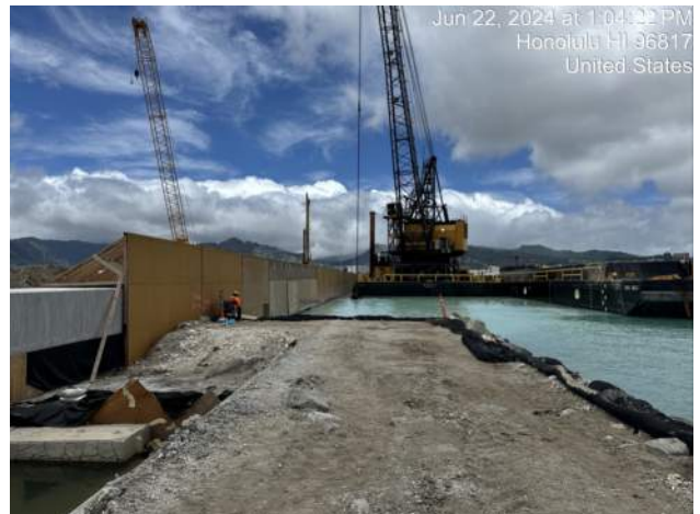
KIWC continued in-water dredging from Sta. 13+00 to 14+00 on Pier 42
