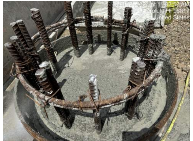
View of shaft 52-A4-36 prior to pulling any casing
