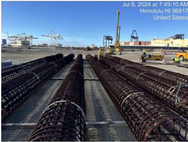
View of CIDH cages for the 36" CIDH shafts staged on Pier 42
