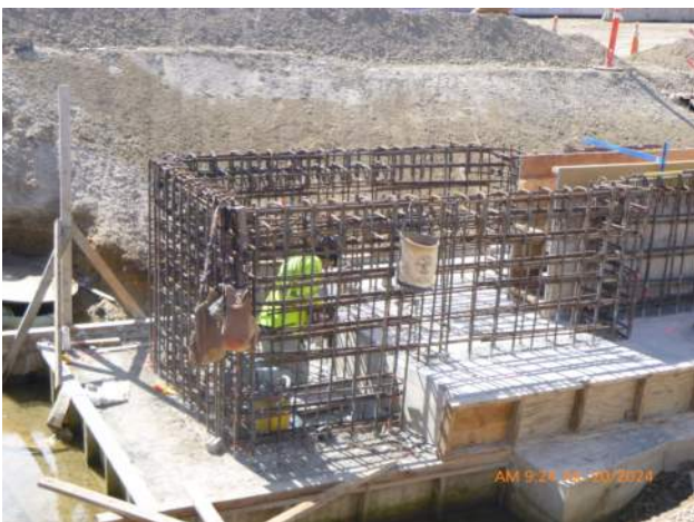
KIWC prepping the TD-3 manhole for formwork installation on pier 41.
