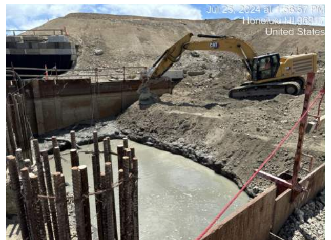
KIWC backfilling the junction structure SOE on Pier 42
