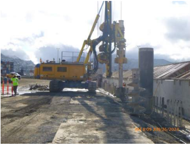
KIWC drilling CIDH shaft 51-A4-36 on pier 42.
