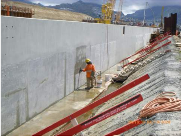
KIWC dry finishing the waterside of capping beam pour #20.
