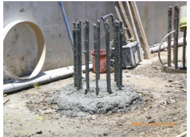
View of concrete in CIDH shaft 37-A4-36 post pour.
