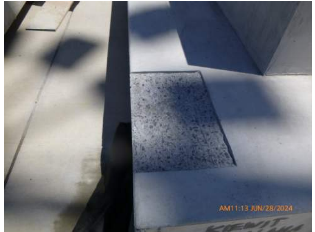
KIWC prepping SDM for spall repair.
