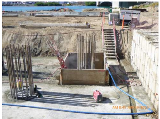
View of trench box around CIDH shaft 05-A1-48A.
