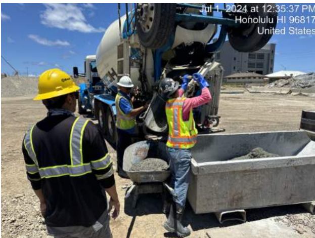
MPE prepping to test truck 1 of the mud mat concrete
