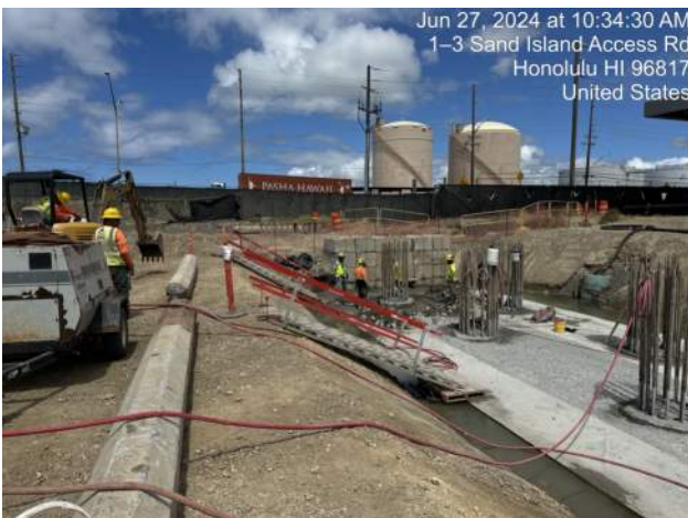
KIWC excavating around shaft 5-A1-48
