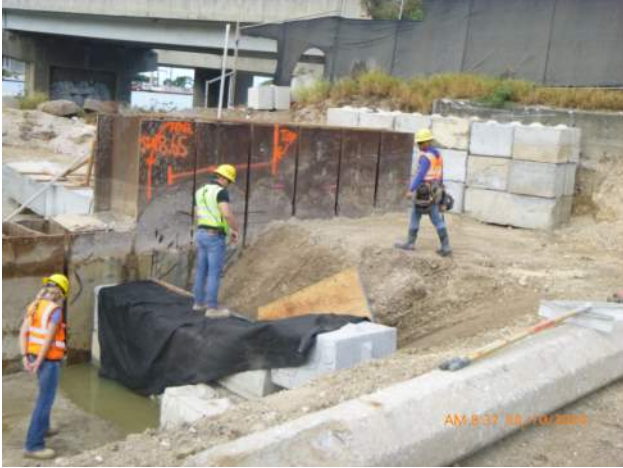
KIWC setting formwork for the capping beam P25 mud mat
