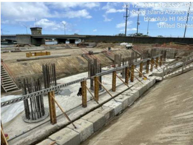
KIWC installing plastic for LSCRB P7 and P8
