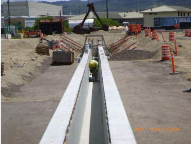
KIWC dry finishing the interior of the pier 41 trench drain.
