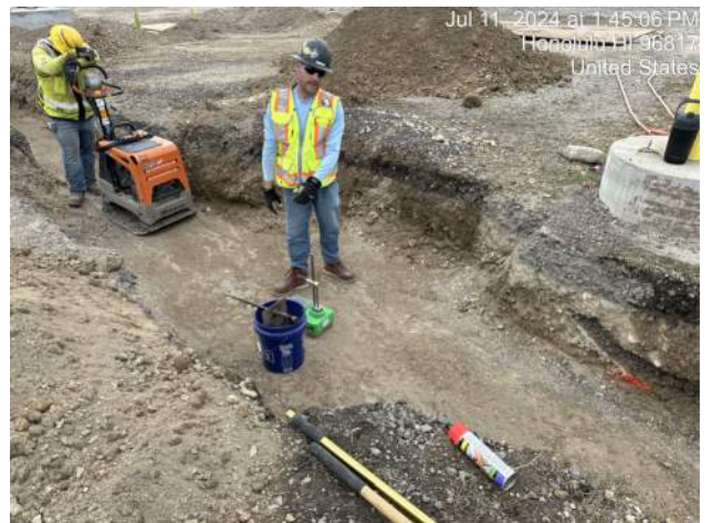
MPE performing compaction testing for lift 1 of the WL-F backfill
