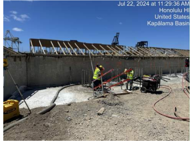
KIWC performing shaft top prep for the WSCRB Sta. 17+00 to 18+50
