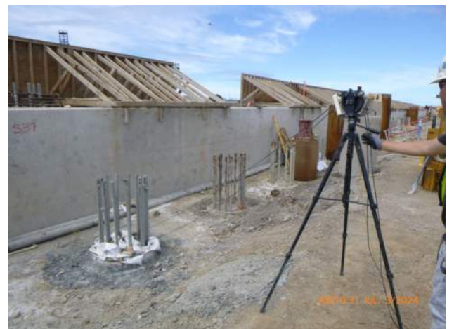
AFT performing CSL testing in 36" CIDH shafts on pier 42.
