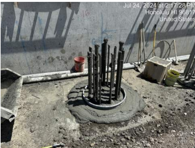
View of completed shaft 16-A4-36
