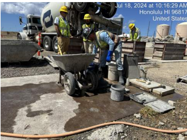
MPE performing concrete testing for the CIDH shafts
