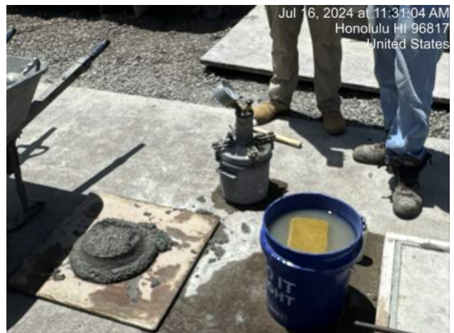
MPE testing concrete for CIDH shaft installation
