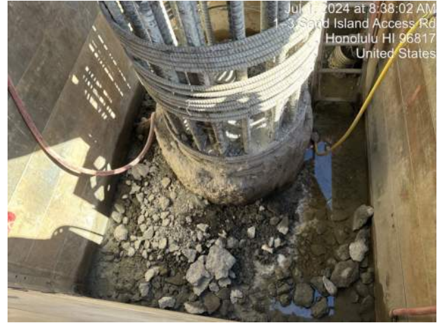
KIWC progress chipping CIDH shaft 05-A1-48 on Pier 43
