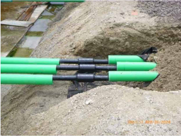
View of installed tie rods on pier 43.
