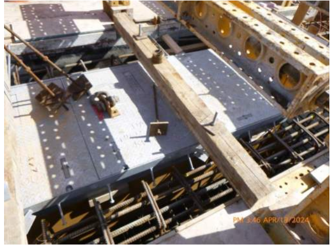
View of shore power vault in capping beam pour #16.
