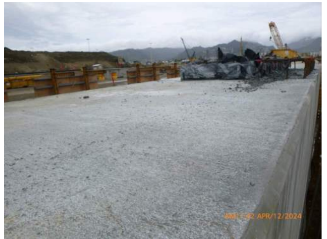
View of the top of capping beam pour #14 on pier 42.
