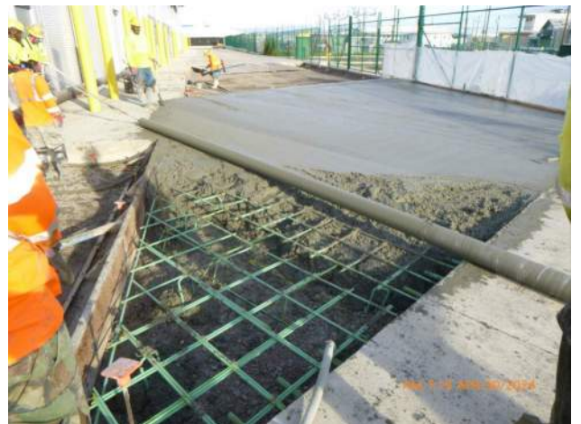
KIWC pouring concrete for PCCP blackout at the maintenance bldg.
