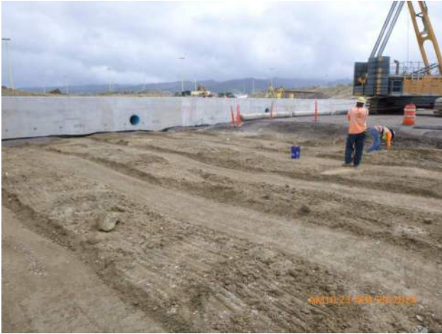
Pier 43: KIWC backfilling over tie rods.
