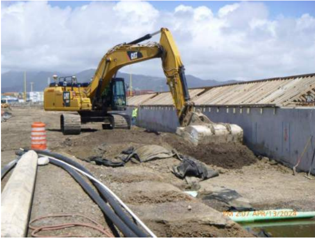
KIWC replacing the backfill along the landside of the capping beam.
