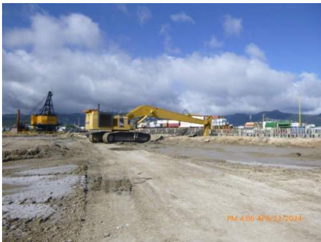
KIWC dredging along pier 41.
