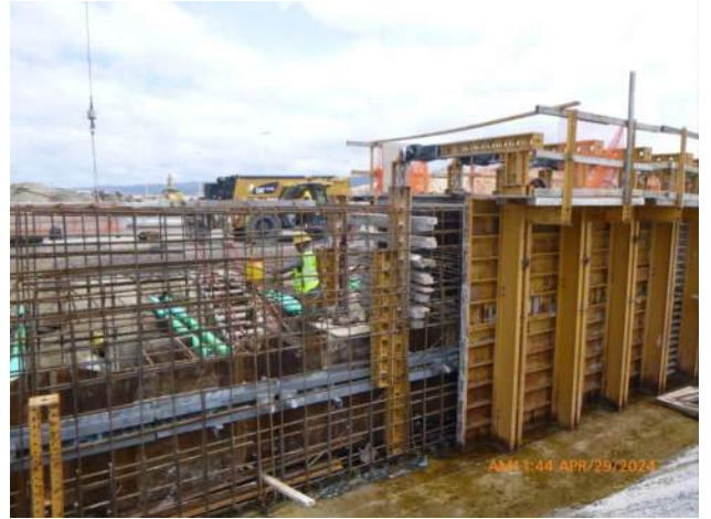
KIWC installing formwork for the capping beam pour #17 bulkhead.
