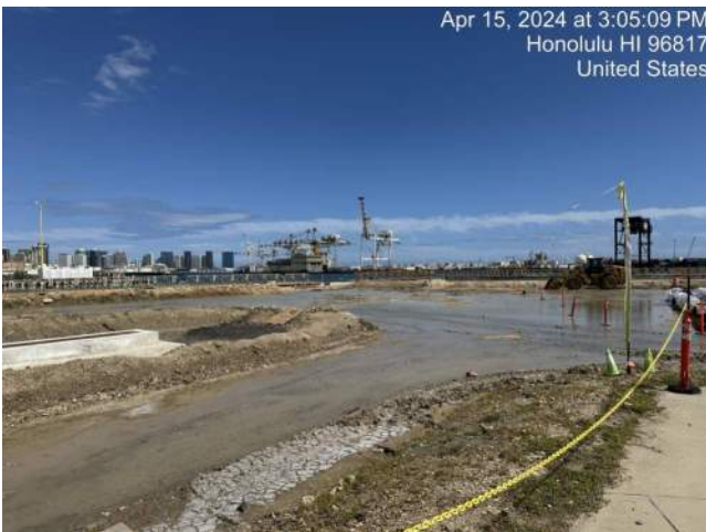
KIWC finished landside dredging for the shift
