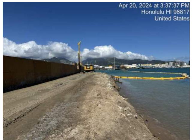
KIWC continued landside dredging using the CAT 349F excavator on Pier 42
