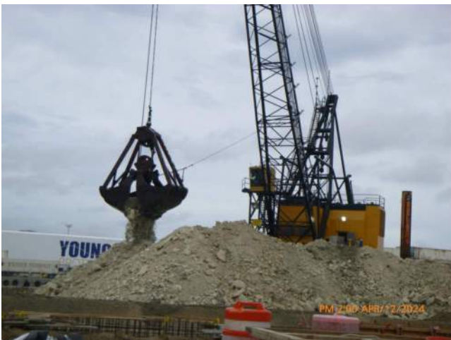
KIWC depositing dredged material onto pier 41.
