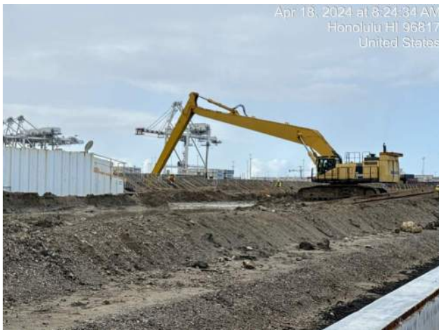
KIWC continued landside dredging on Pier 41
