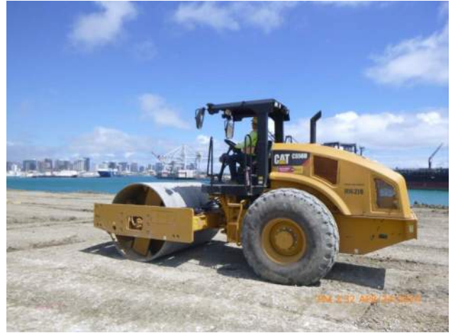
KIWC rolling lift 16 of the snug harbor surcharge.
