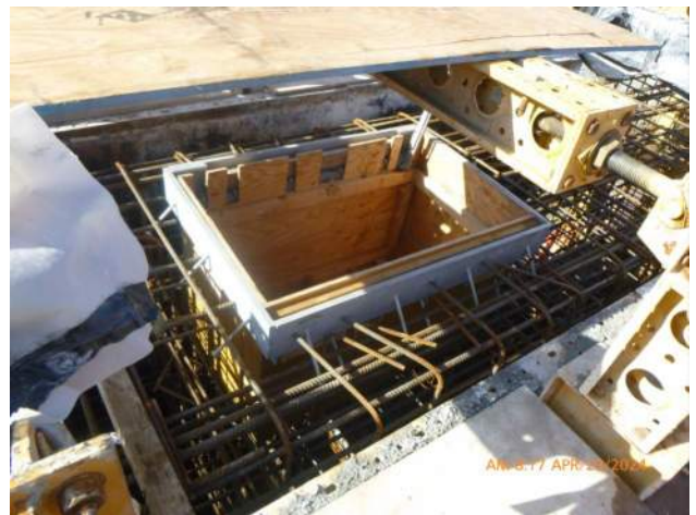
View of the water vault in capping beam pour #17 on pier 43.
