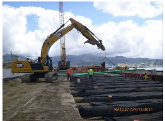
KIWC setting tie rods on pier 43.
