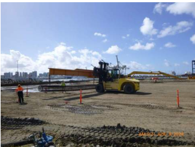
KIWC moving 36" CIDH rebar cages to the staging area on pier 42.
