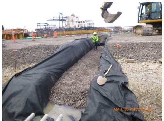
KIWC installing 3b stabilization layer beneath the tie rods.
