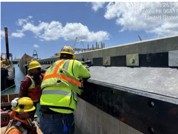
KIWC bridge and marine fastening fenders using 3/4 drivers
