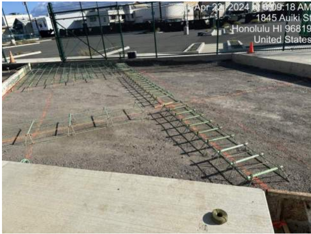
View of the north breakout area of the maintenance building area
