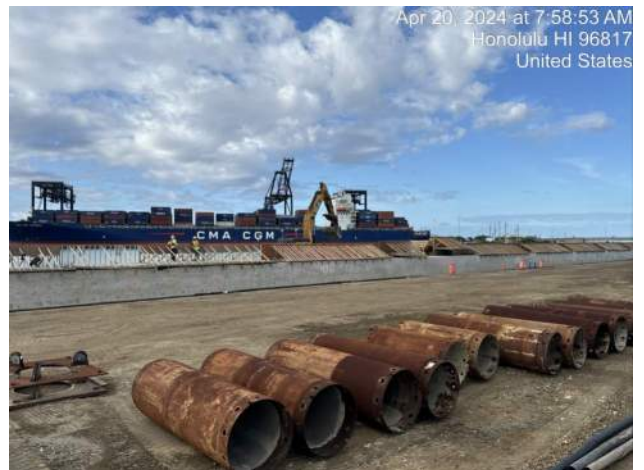
KIWC continued landside dredging on Pier 42 using the CAT 349F excavator
