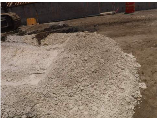
Pier 42: Drill spoils consisted of light brown coral sand and gravel from CIDH #40-A4-36 at 52' bgs
