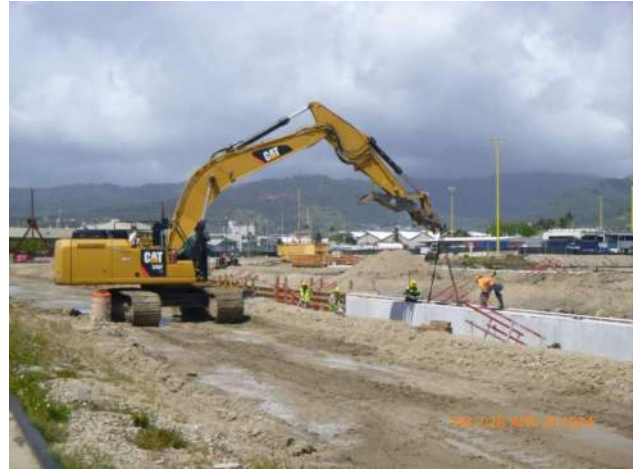
KIWC stripping formwork from around TD-3.
