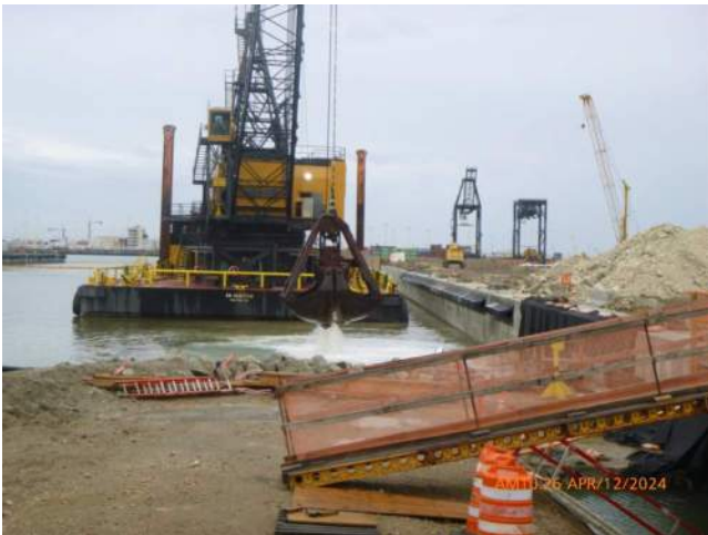
KIWC dredging along the pier 41 capping beam.
